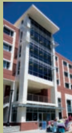
Dragon Hall, SUNY Cortland's 18th residential building, officially welcomed 229 students this fall, offering a range of modern amenities and impeccable “green” credentials. Features in the $22 million structure include rooftop solar panels, environmentally sensitive lighting and a new type of heat-conserving insulation.
